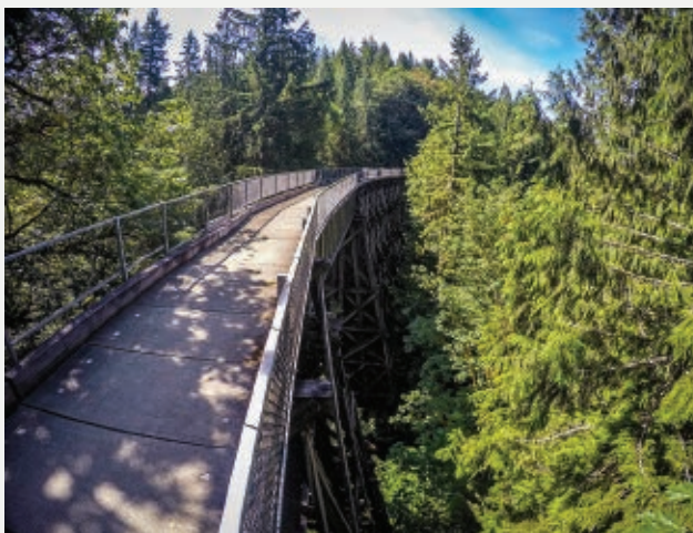
Snoqualmie Valley Trail Tokul Trestle
